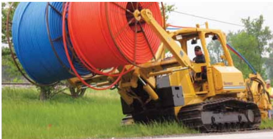
Tharp Brothers work on the fiber optic route outside of Colchester.
